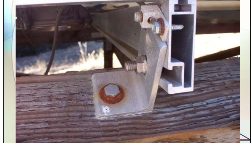
How about those Cad-plated fasteners and Tek screws to rails
